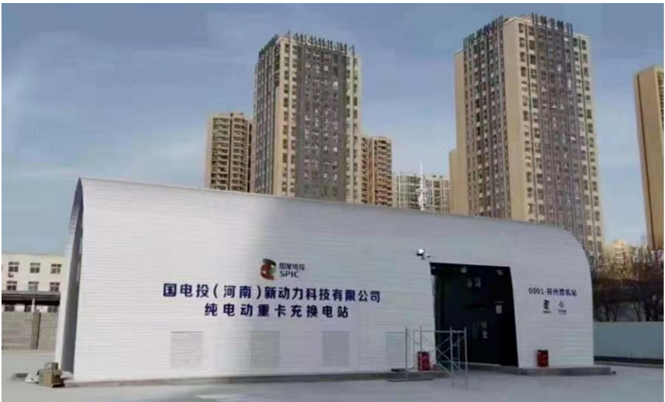
Figure 30: EHT battery-swapping station in Zhengzhou, Henan province.
