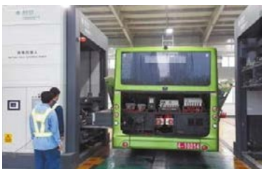
Figure 12: Side battery mount
